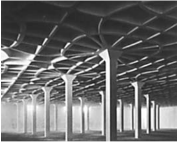
Fig. 5: The Gatti wool factory ceiling structure
